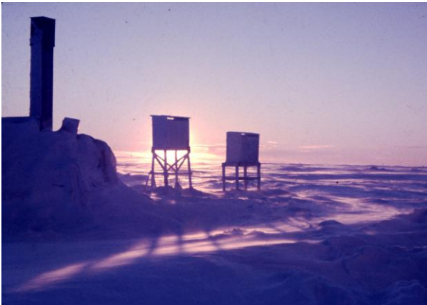
Figure 8: The theodolite post and weather "beehives" at Ice Station T-3, September 1963. The blowing snow in the foreground is due to increasing wind, which later became a blizzard (JLBerry)
