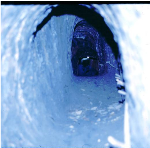
Figure 10: Cross-cut at Nkana, Zambia, 1968. The tunnel is 2' wide, 3' high, and 25' long. The tape pegged to the wall enables the geologist to describe the rocks and locate their contacts. The sampler, in the distance, will follow the geologist, cutting a channel sample along the tape( JLBerry).
