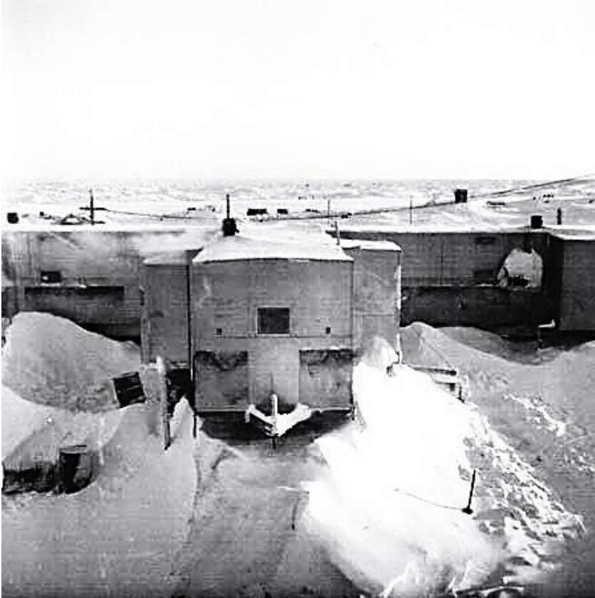
Figure 2: The Mess Hall at T-3 in 1961. This building burned down with a loss of life in 1962 after fuel pumped from the bilges of visiting icebreaker Northwind was used in the furnace. The fuel contained seawater, which put the furnace out, but the burner remained hot enough to explosively ignite the next “slug” of fuel to reach it. (Courtesy web-site kf3aa)
